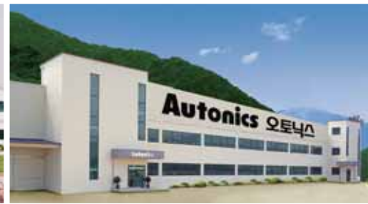
Headquarters / Factory (Yangsan, Korea)
